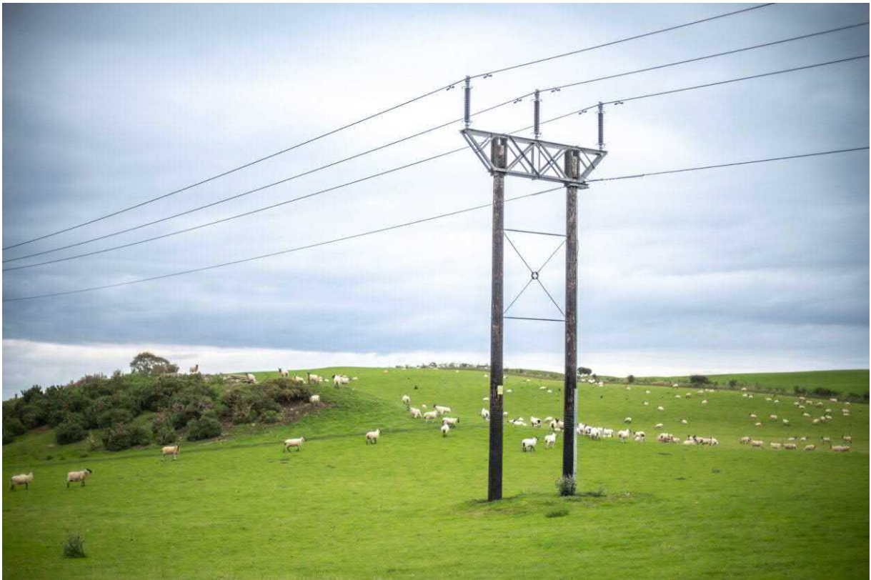
Figure 2.1: Typical intermediate 'H' pole
