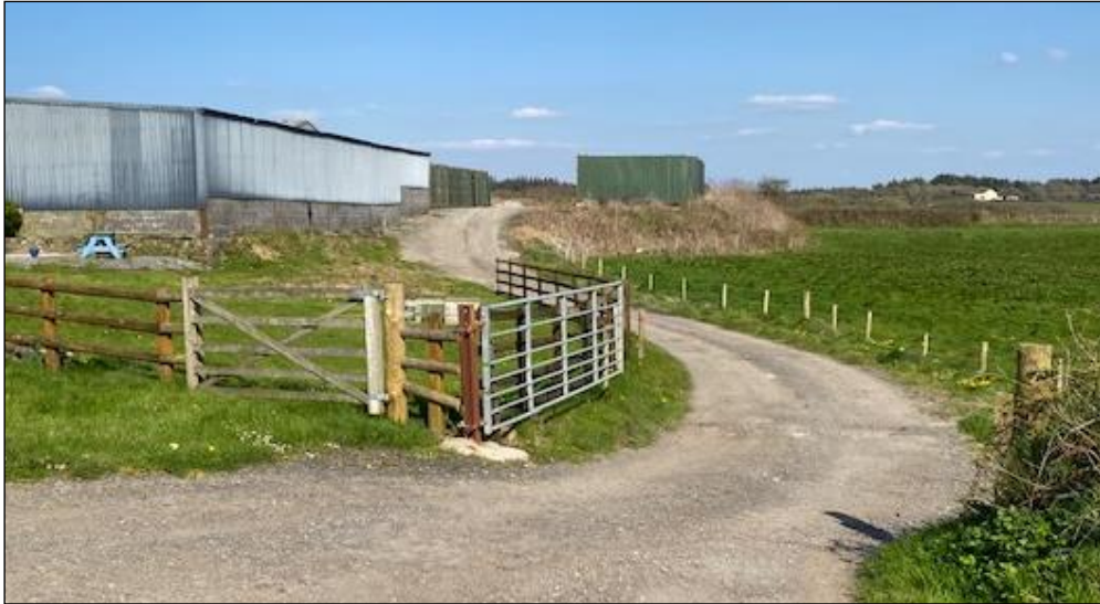
Photograph 4 – view from farm gateway looking along track to compound yard and containers against backdrop of tall portal framed sheds
