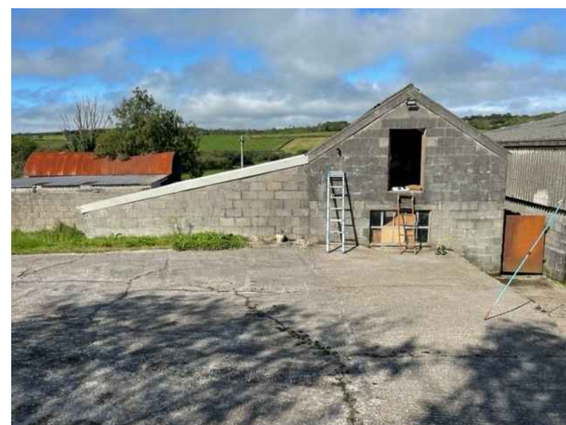
Rear elevation Picture
